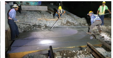
Construction of the beam bearing of the First Minxiong Bridge
