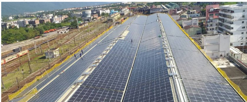
PV modules on Hualien workshop's rooftop (Courtesy of Li R Shin Corporation)
