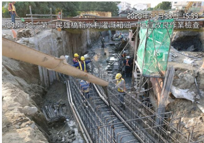
Construction of new culvert of First Minxiong Bridge
