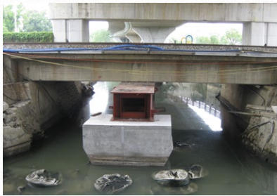
Erection of east-west support steel beam
