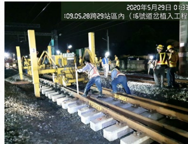
Re-laying of turnouts of the First Minxiong Bridge
