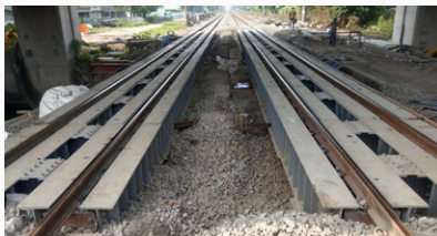
Construction of East and West Main Line beams
