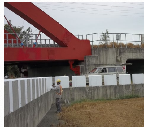
Guardrail block painting
