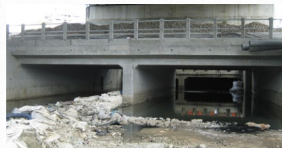
Completion of RC culvert construction of the main works
