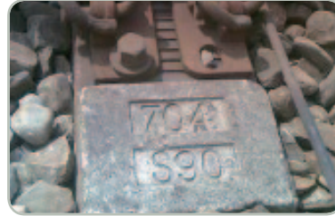
PC 接頭大枕托接 PC supported joint on the tie
