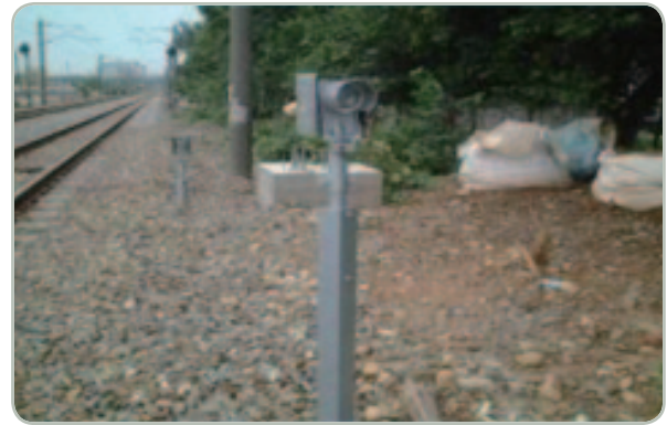
平交道障礙物自動偵測設備 Crossing Obstacle Automatic Detection Equipment
