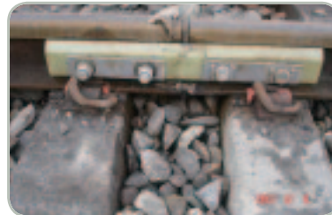
塑鋼絕緣接頭以 PC 軌枕懸接方式裝設 Insulated plastic steel joint installed with PC tie suspension
