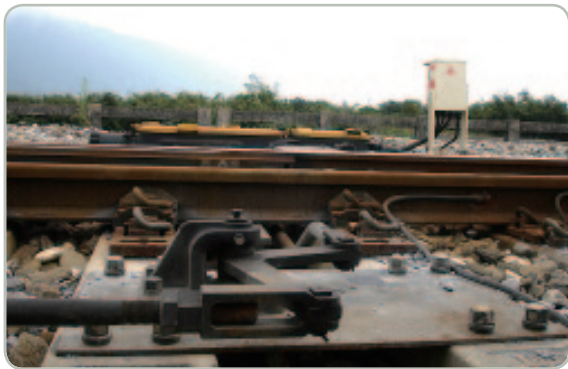
實際安裝於嘉新站南端 #12PC 枕道岔 #12 turnout supported by PC ties installed at the south of Chiaxin Station
