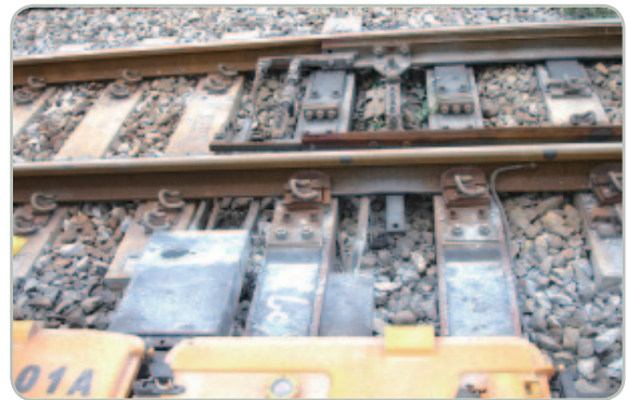
嘉新站南端 #12PC 枕道岔 (俯視圖) #12 turnout supported by PC ties installed at the south of Chiaxin Station (the vertical view)
